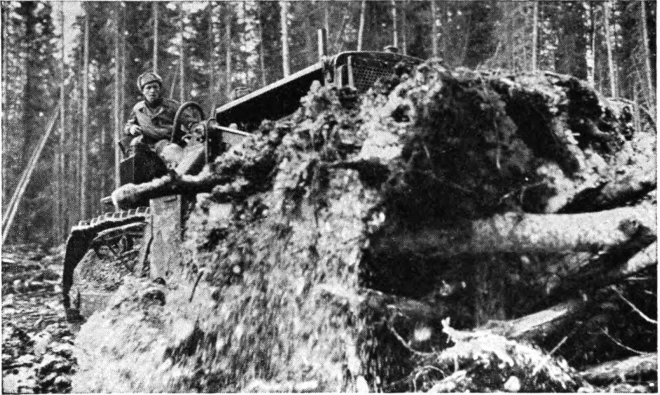
Figure 47. Removing cleared material from site.
